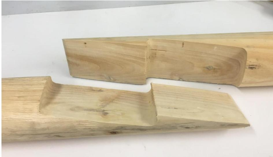
CNC routed Hooked scarf Joint
